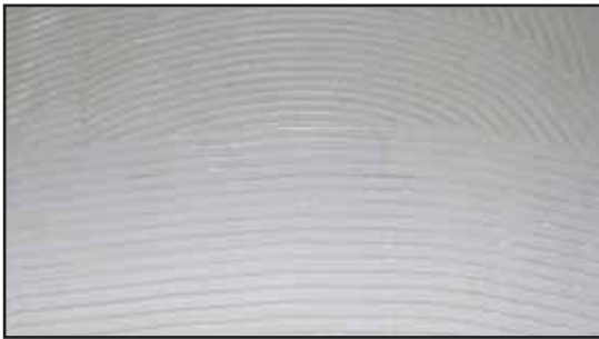
Example of properly troweled adhesive application
